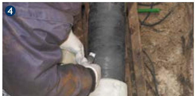
4 Wind adhesive tape around the ends of the Pipecast tape in order to press it firmly on to the pipe.
