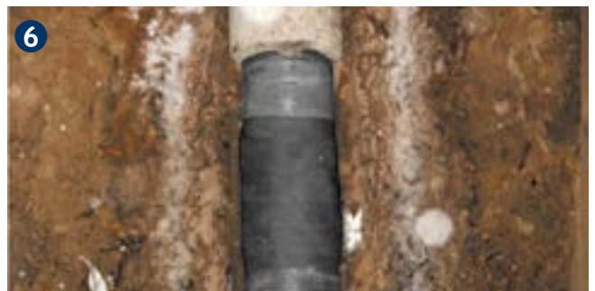
6 Pipecast after pressing.
