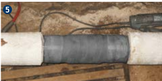
5 Allow the Pipecast to cure for 20-30 minutes at 23 °C. It is ready to be buried after in approx. 1 hour.
