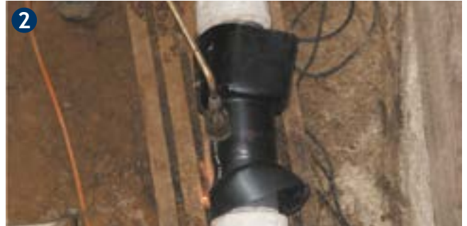
2 Installing the shrink sleeve
