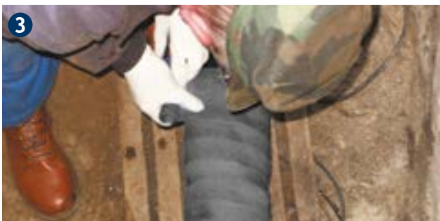
3 After saturating with water, wind the Pipecast tape around the pipe with a minimum of 1 x 75% (4 layers) overlap.
